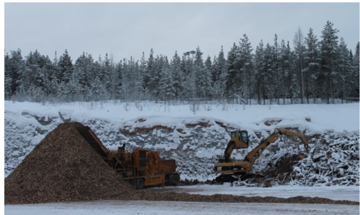
Figure 1. Stump crushing at a terminal
